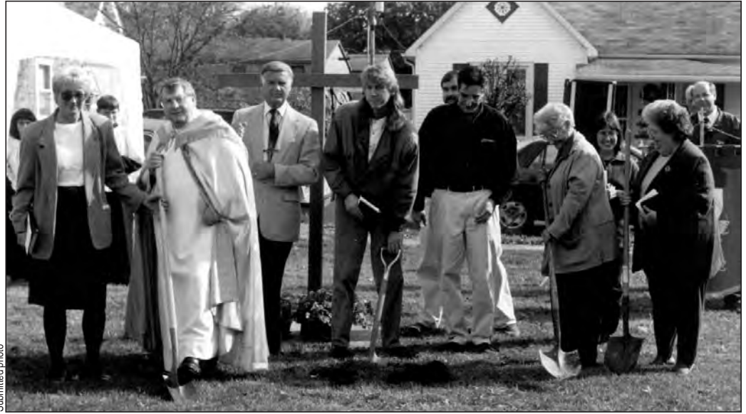
Father Paul M. Dede, pastor, along with members of the St. Jude Parish Council, the Building Committee and parishioners, gathered for Mass and the Rite of Ground Breaking and blessing of the construction site of St. Jude the Apostle Parish's new church building Oct. 25 in Spencer.
