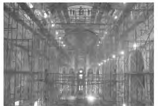
Scaffolding now fills the church interior.
