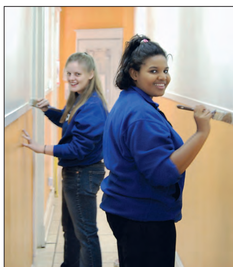
Bishop Chatard freshman Katie Armstrong, left, and sophomore Shari Bailey paint the interior of a home being restored by "Rebuilding the Wall," an organization that restores vacant homes for low-income families.
